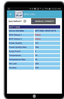
Replace as no protection is left
